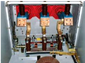
ANSI Standards – Type VCP-W Vacuum Circuit Breaker Rated on Symmetrical Current Rating Basis ❶
